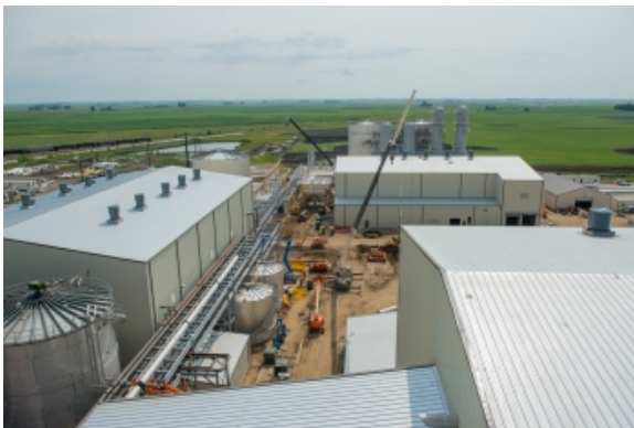
POET-DSM's Project LIBERTY opened in September becoming the nation's first commercial-scale cellulosic ethanol plant to use corn waste as a feedstock. | Photo courtesy of POET-DSM
