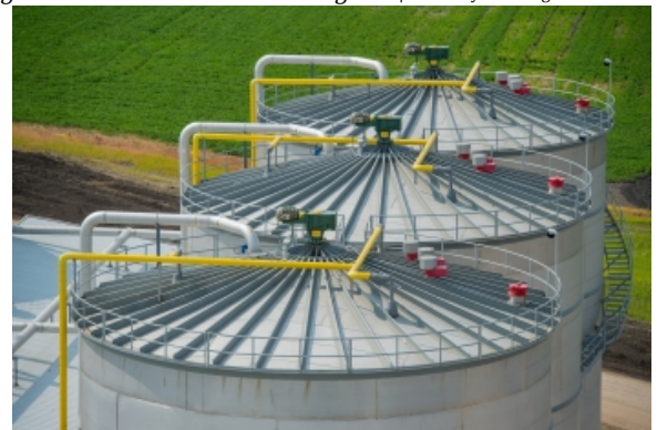
Fermentation tanks at POET-DSM's Project LIBERTY biorefinery in Emmetsburg, Iowa. The biorefinery uses a biological process to convert post-harvest corn stover into biofuel. | Photo courtesy of POET-DSM
