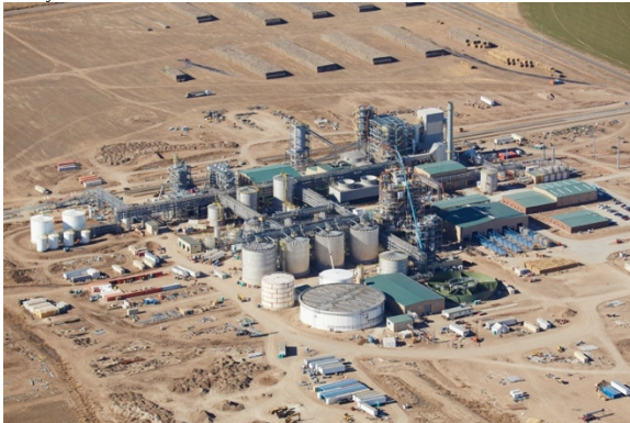
The Abengoa Bioenergy Biomass of Kansas facility has the capacity to convert up to 325,000 dry tons of agricultural residues, including corn stover, in to 25 million gallons of cellulosic ethanol each year. | Courtesy of Abengoa
